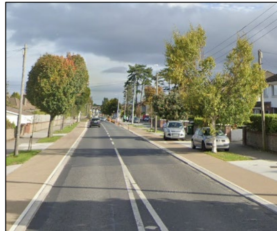
Figure 5-2: Example of a Segregated Cycle Track
