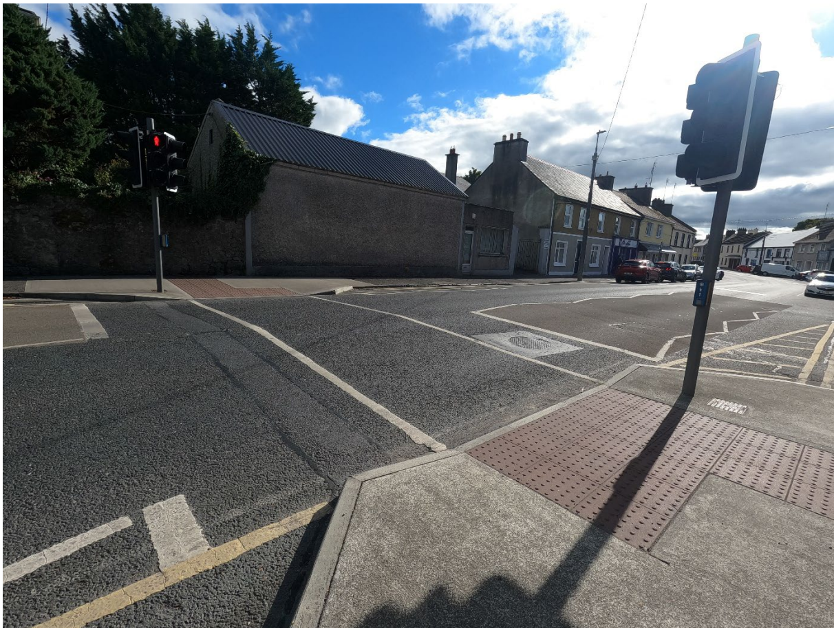
Figure 3-22: Church Road Signalised Crossing
